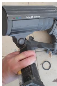
CAMERA DE SURVEILLANCE
